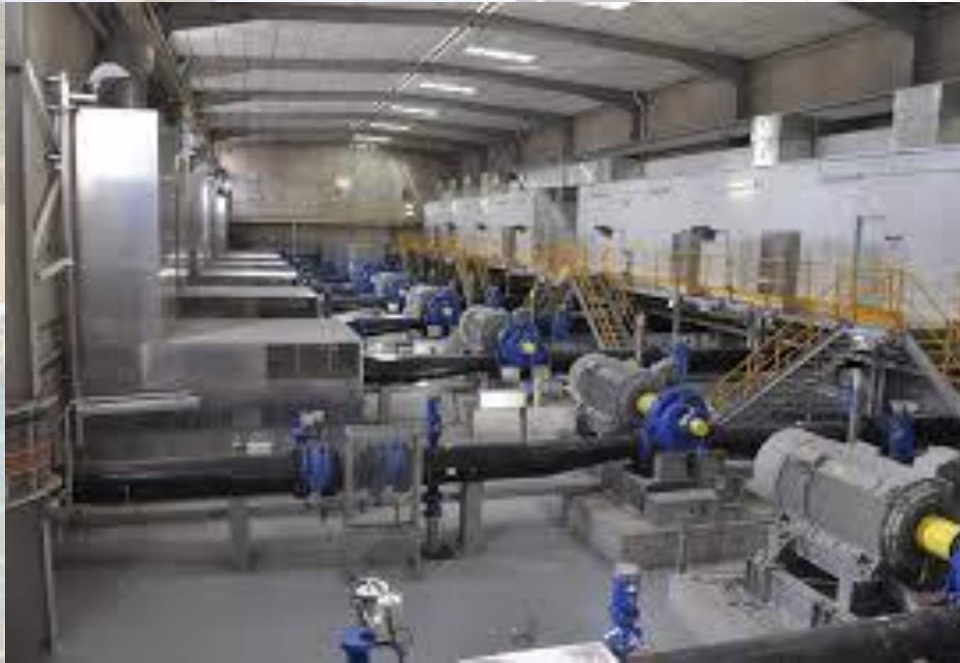
Desalination Plant, Basrah, Iraq.
