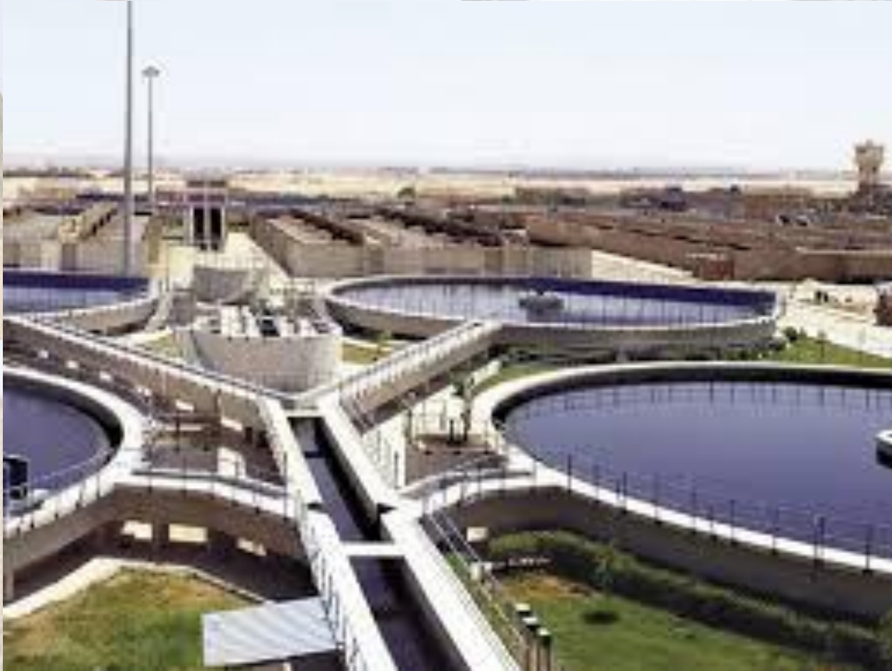
Water Treatment Plant Sharkeya Governorate
